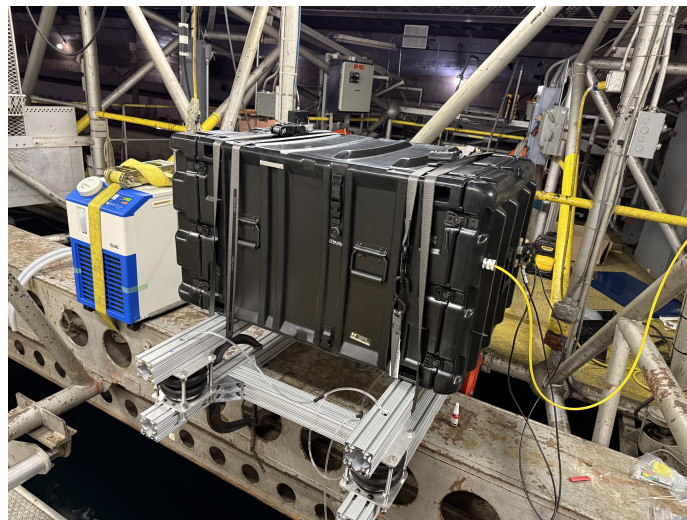
Figure 6. Climate-controlled enclosure housing the laser mounted to the central strut of the carriage. The yellow cable exiting the box on the right of the image is the 30-m-long optical fiber used to deliver laser light. A chiller with lines going to the laser can be seen on the left of the image. The housing is mounted onto a vibration-damping rack.
